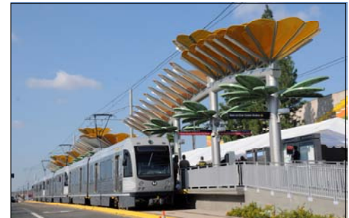
The Eastside extension of the Gold Line (light rail transit) opened in November 2009 with an amazing safety record with no lost time due to injuries during construction.
